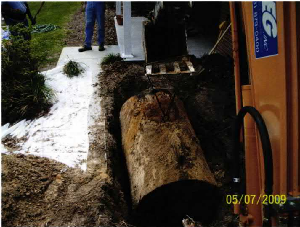
Picture 1: UST 1003Bobwhite Drive being removed from the excavation.
